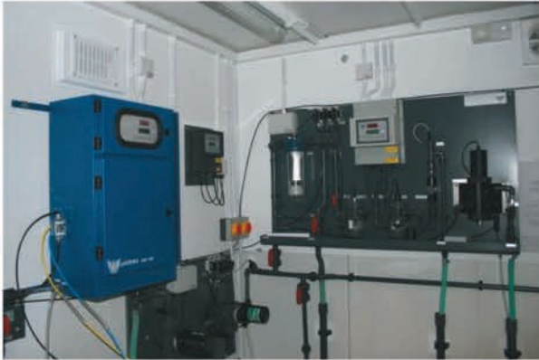
River & Potable Water Monitor
